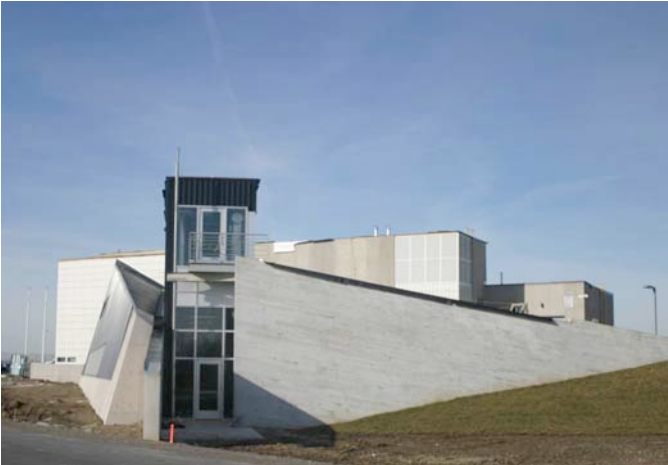
GTAA Fire training facility - photo courtesy of Kleinfeldt Mychajlowycz Architects
